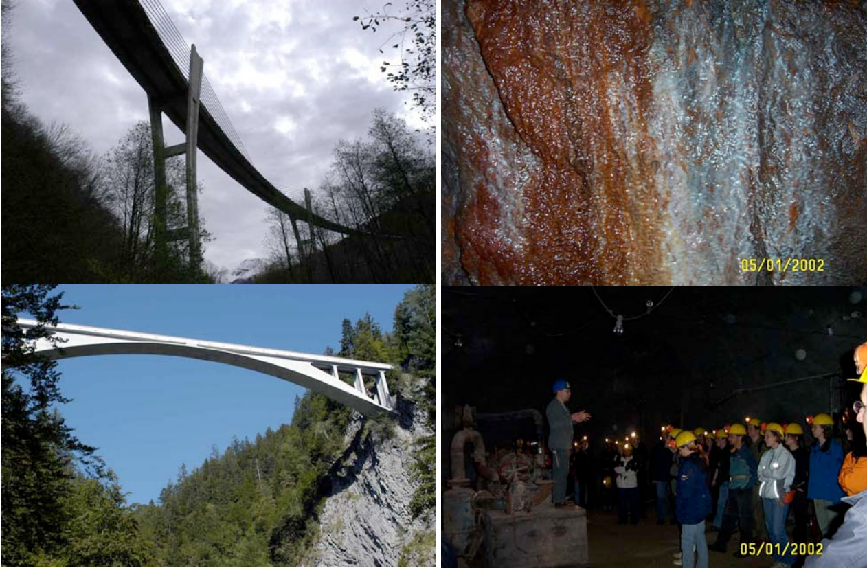
Sunniberg bridge (Klosters) Salginatobel bridge (Schiers)
